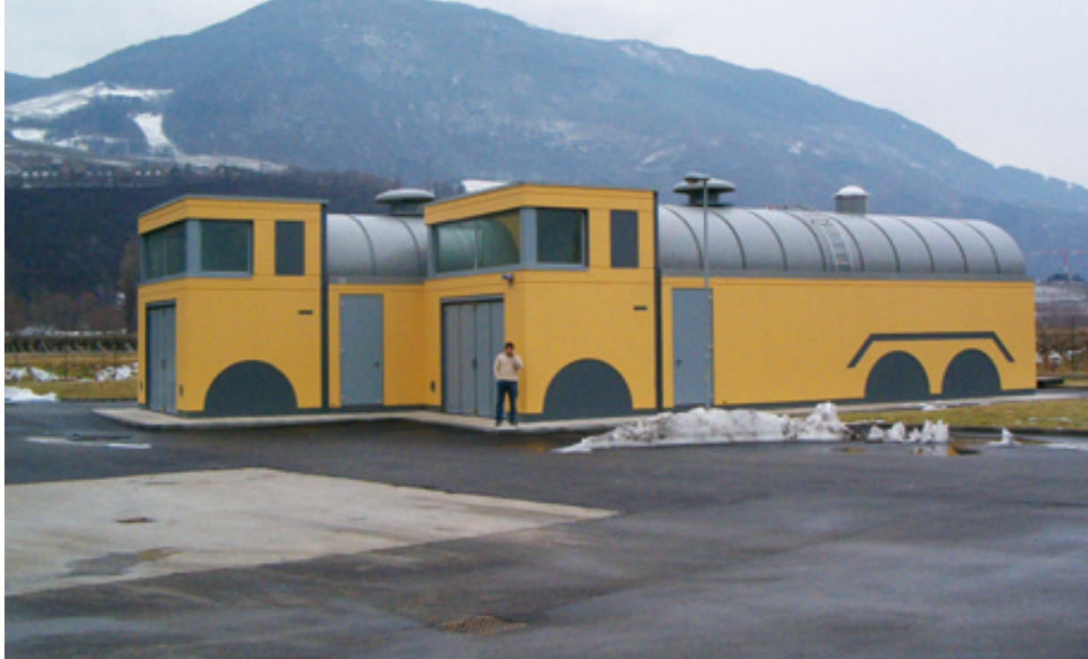
Filtration plant coverings – Mezzocorona (TN)
